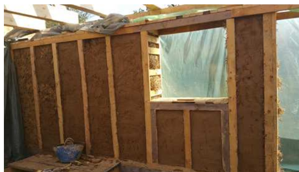
Fig.4. Wall under construction, using straw bales infill walls, in Cluj County, Romania.
