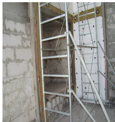
Fig. 3. Basalt mineral wool edging of the perimeter of the fire compartment and next to the floor on the 1st floor
