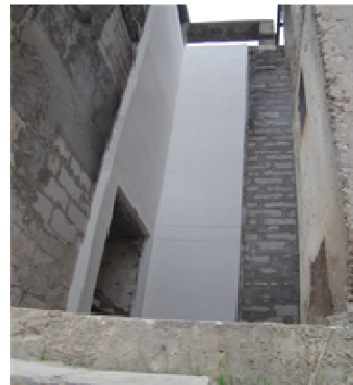
Fig. 6. ETICS system ready for fire testing
