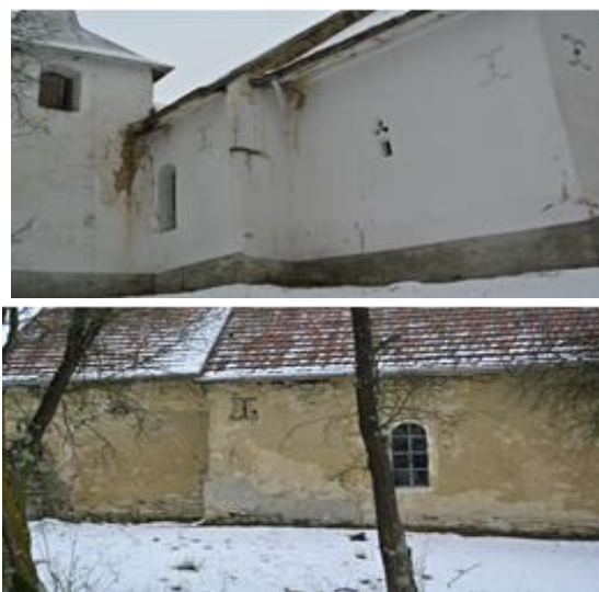
Fig. 7. North facade and south facade
