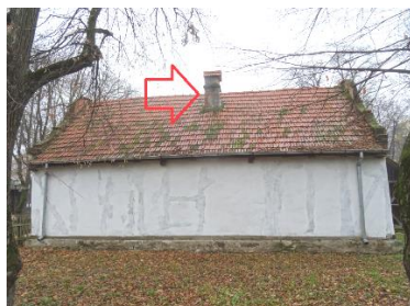
Fig. 12. Clay brick chimney
