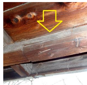
Fig. 15. Cross-halving of the beams
