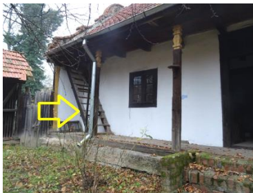
Fig. 11. Stairs to the attic
