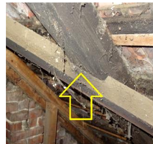
Fig. 14. Cross-halving of the roof structure
