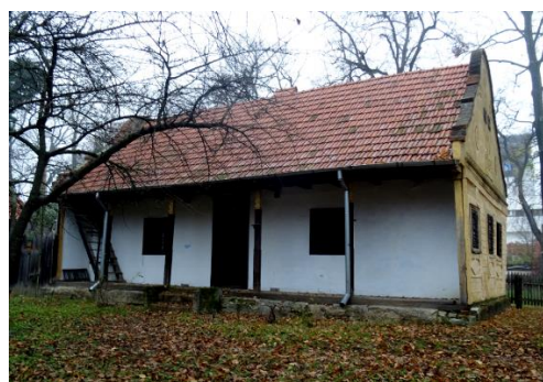
Fig. 7. Front side of the house
