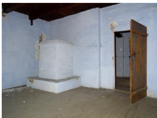
Fig. 5. The flooring made of processed planks
