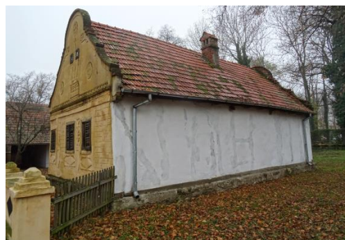
Fig. 8. Front side of the house
