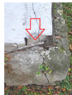
Fig. 16. Cross-halving of the sill plates at corners
