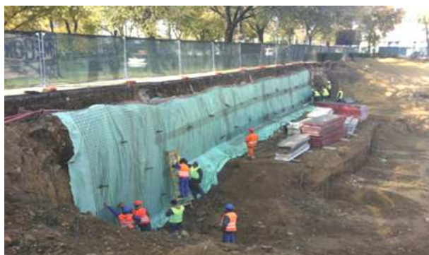
Fig. 4.a. Targeting the walls of an anchor excavation and protecting it with shotcrete. Palace of Justice in Iasi (PROXEROM, 2019)
