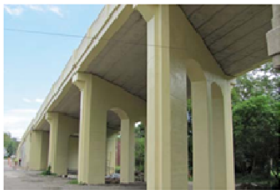
Fig. 4.c. Blaine Hill Viaduct 40 Ohio (US) built in 1933, with a 307m (307m) length of concrete (Pinney, 2012)
