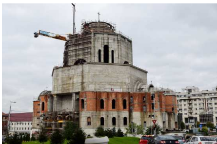
Fig. 3.a. The Greek-Catholic Cathedral in Cluj-Napoca, with a height of 48 m, to which the shotcrete was sprayed over the brick masonry (Radio Cluj, 2019)
