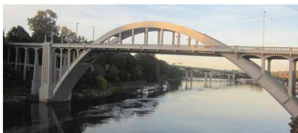
Fig. 4.b. The Oregon Bridge over the Willamette River, rehabilitated in 2012 (Marcus, 2014)
