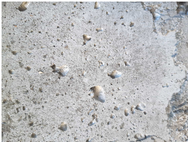
Fig. 3. Example of porous concrete surface
