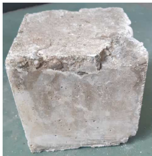
Fig. 7. Example of broken edges
