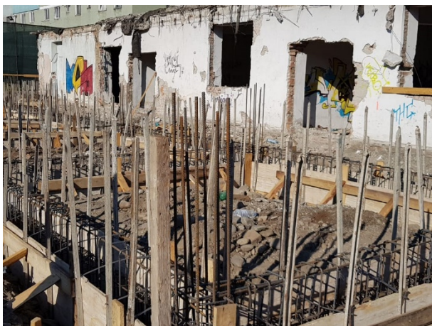
Fig. 5. Current stage of the rebuilding phase
