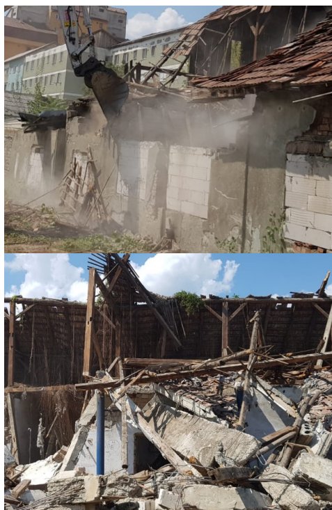
Fig. 2. Aspects from the demolition process
