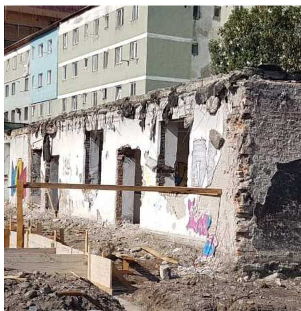
Fig 3. Part of the building without the old roof
