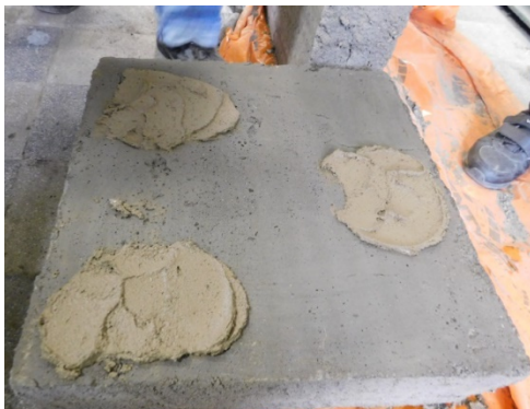
Fig. 4. Placing the composition on the earth wall
