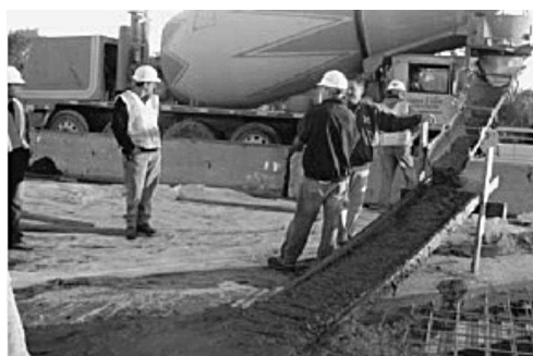
Fig. 7. In situ casting of ECC M45 with self-compacting fresh state behaviour (Li, 2008)
