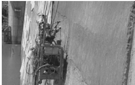
Fig. 9. Spraying ECC mix for large surface repair techniques (Li, 2008)
