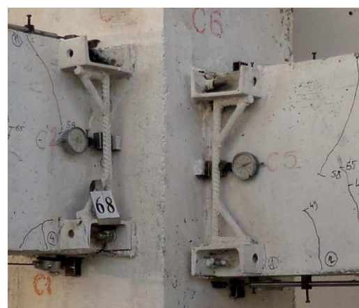
Fig. 12. SH-FECM placed at beam to column interface (Baeră et al., 2016a)
