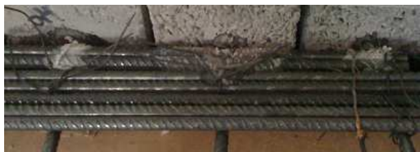
Fig. 16. Deposits of salt crystals
