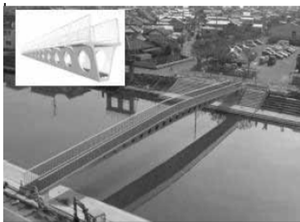
Fig. 4. Pedestrian bridge Sakata Mirai (Japan, 2002) [7]
