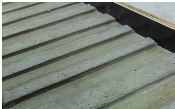
Fig. 4. Precast slabs with stepped top surfaces
