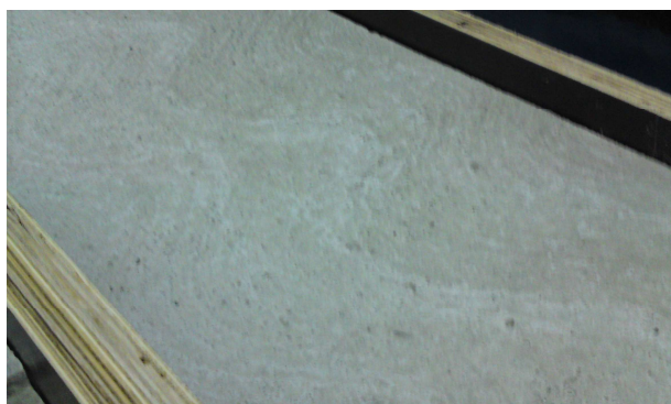
Fig. 3. Precast slabs with broom-swept tracks
