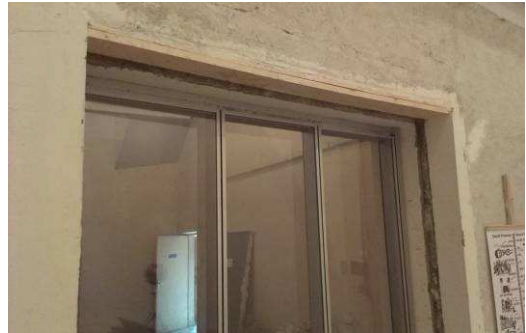
Fig. 5. Detail of the positioning of the partition wall system DUO twinglass type (3.1.3-81-6) in the airborne sound insulation stand
