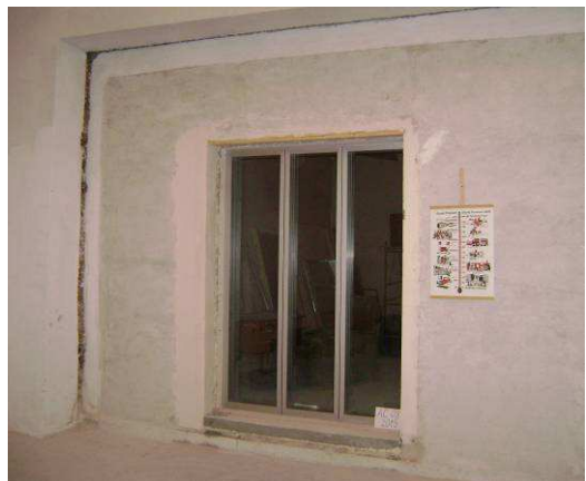
Fig. 6. Detail of the positioning of the partition wall system DUO twinglass type (4-83-6), in the airborne sound insulation stand
