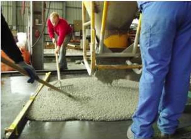
Fig. 7. Placing of self-compacting concrete for the filigree slab. Gelissen Precast Factory (Holloweg)
