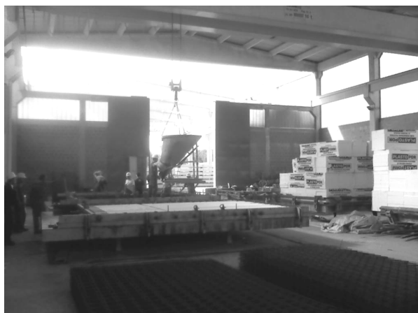
Fig. 5. Production of floor slab elements
