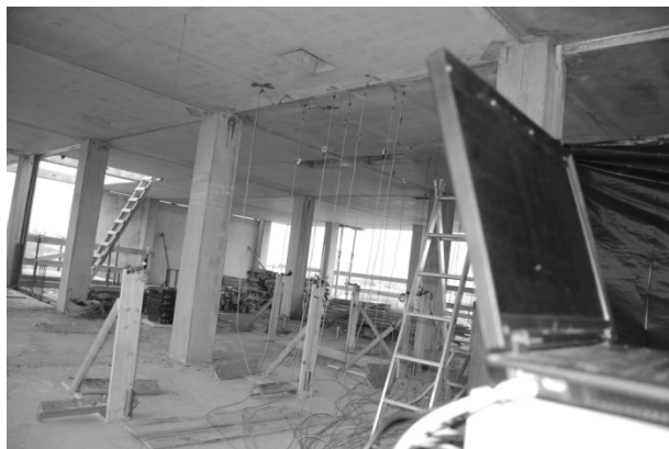
Fig. 8. Load testing in progress
