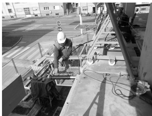
Fig. 4. Prestressing in progress
