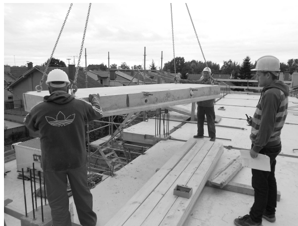
Fig. 6. Assembly of cantilevered floor slabs
