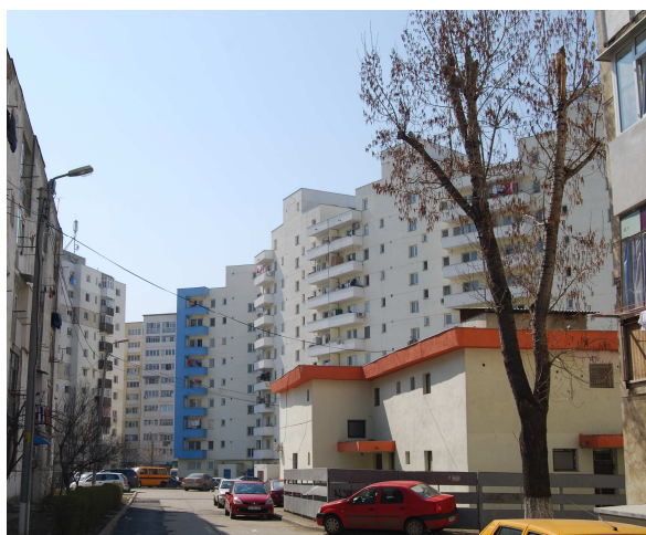
Figure 2. Thermal rehabilitation of buildings – facade interventions
