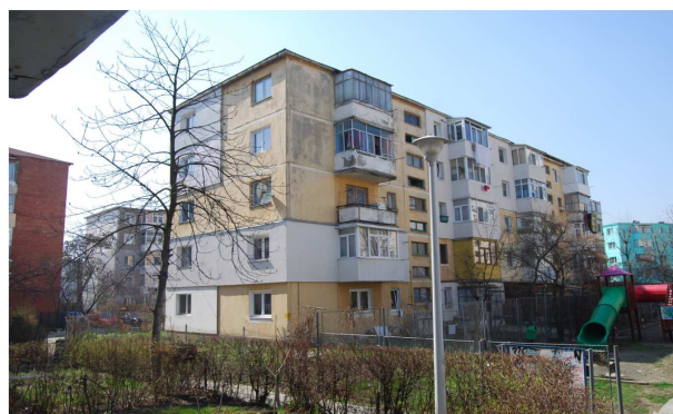
Figure 1. Chaotic thermal rehabilitation interventions carried out on a collective housing building made of large panels.
