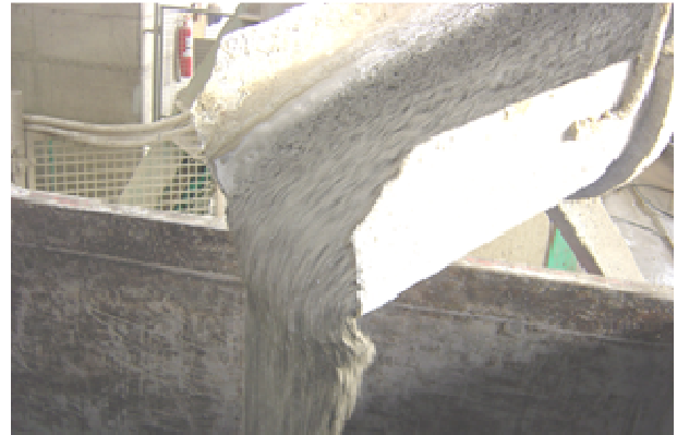
Fig. 4. Image taken during the casting of structural elements
