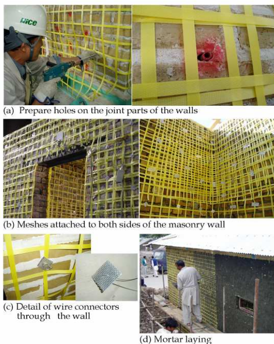
Fig. 1. PP-band retrofitting method
