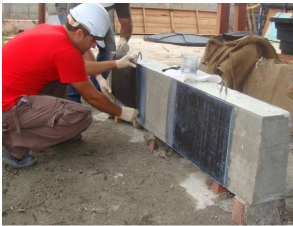
Fig. 2. Deep beam strengthening by CFRP using wet lay-up system
