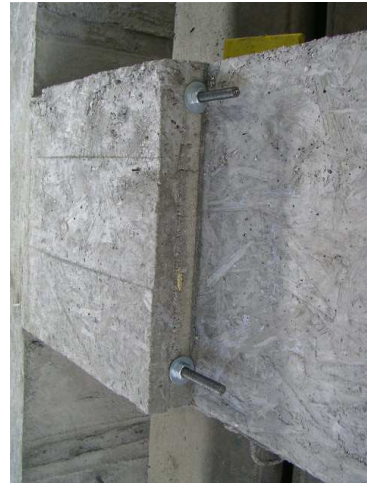
Fig. 2. Fixing of non-adherent special reinforcement
