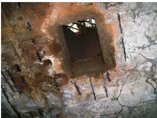
Figure 11. Bottom view of the slab in the access of rainwater drainage
