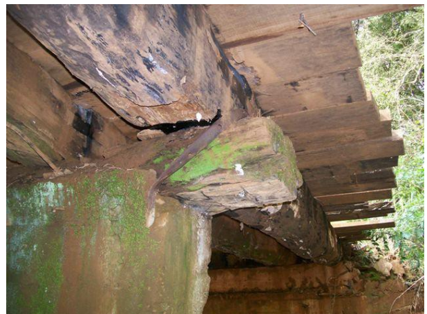
Figure 22. Cantilevered crossbeam to support beams
