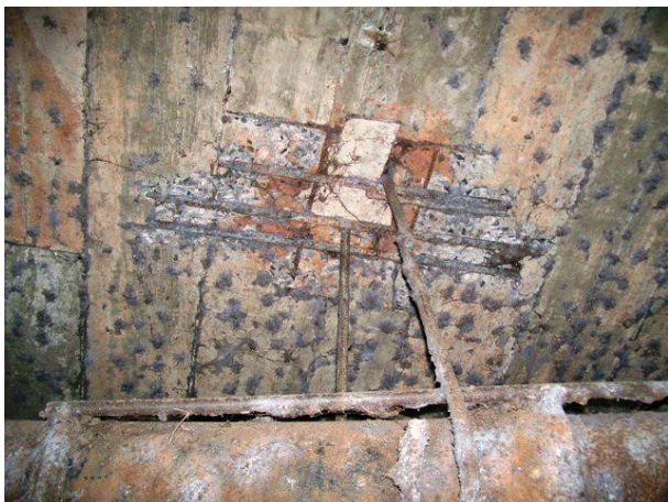
Figure 10. Detail of fixed pipes in the slab of the bridge
